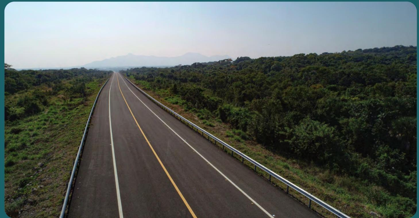
In an effort to improve the mechanical characteristics of bituminous mixtures and prolong the working life of road surfaces, ME Concessions, ME Global and MEEC undertook a pilot project in the Douro Interior subconcession. This project involved incorporating rubber from used tyres into
