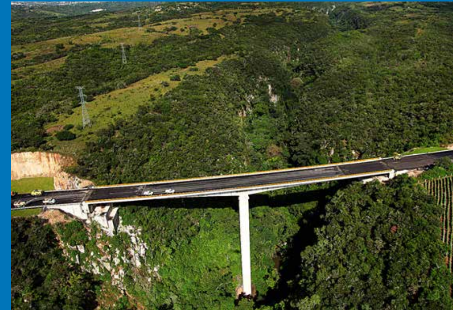
Puente Cimarron-Xalapa, México Cimarron-Xalapa Bridge, Mexico
